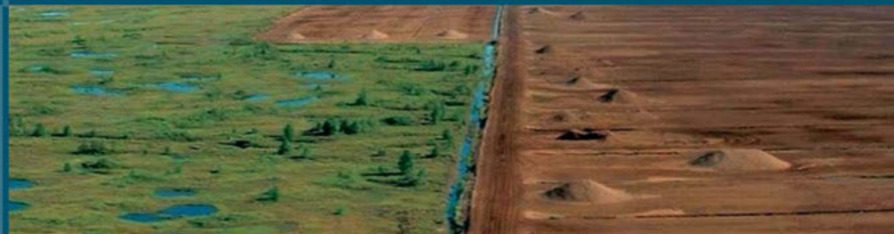
A bog wetland being stripped for peat.
